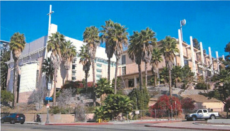
The former headquarters of the Los Angeles Metropolitan Water District on Sunset Boulevard. (Michael Owen Baker / For The Times)
